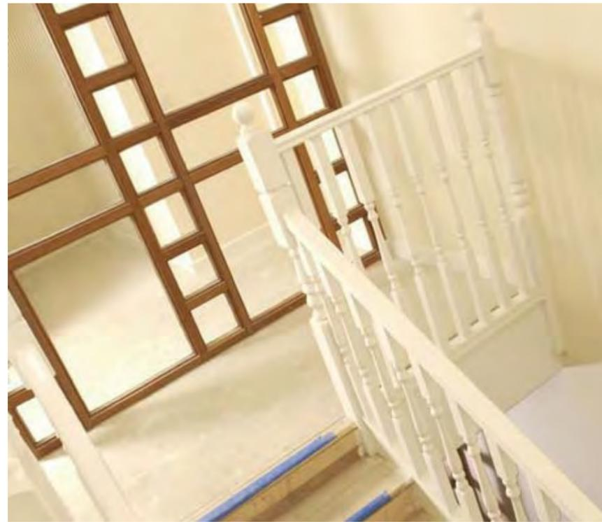
FIG 5. STAIR COVERING AND INDEPENDENT CEILING WITH SOUND ABSORBING MATERIAL
