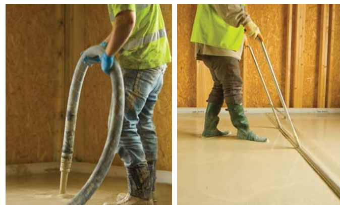
6. 40mm minimum SoundBar Gyvlon screed is then poured and levelled.
