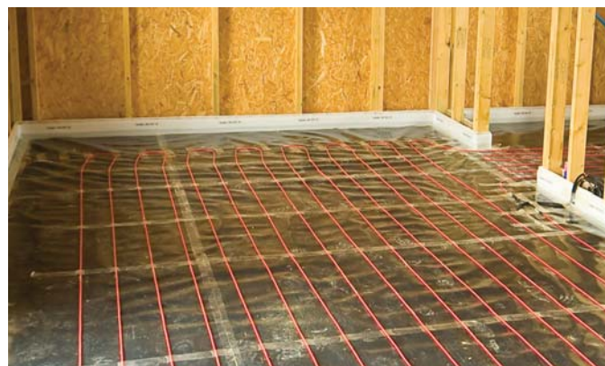
5. Install under floor heating at this point if required*.
