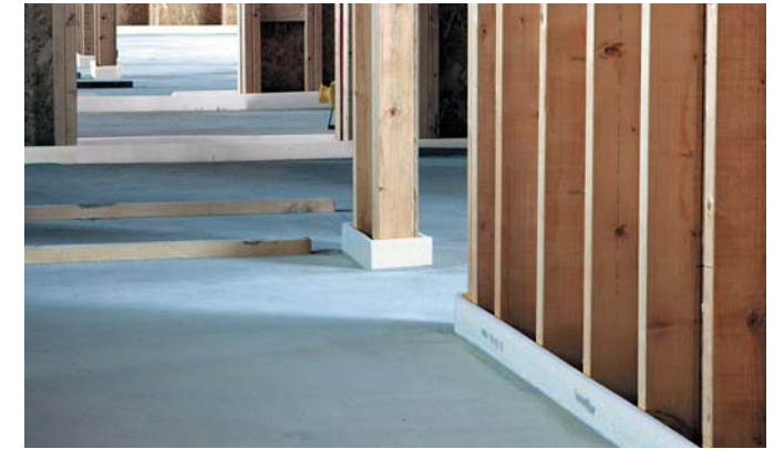
8. 48 hours later screed is dry enough to walk on.
